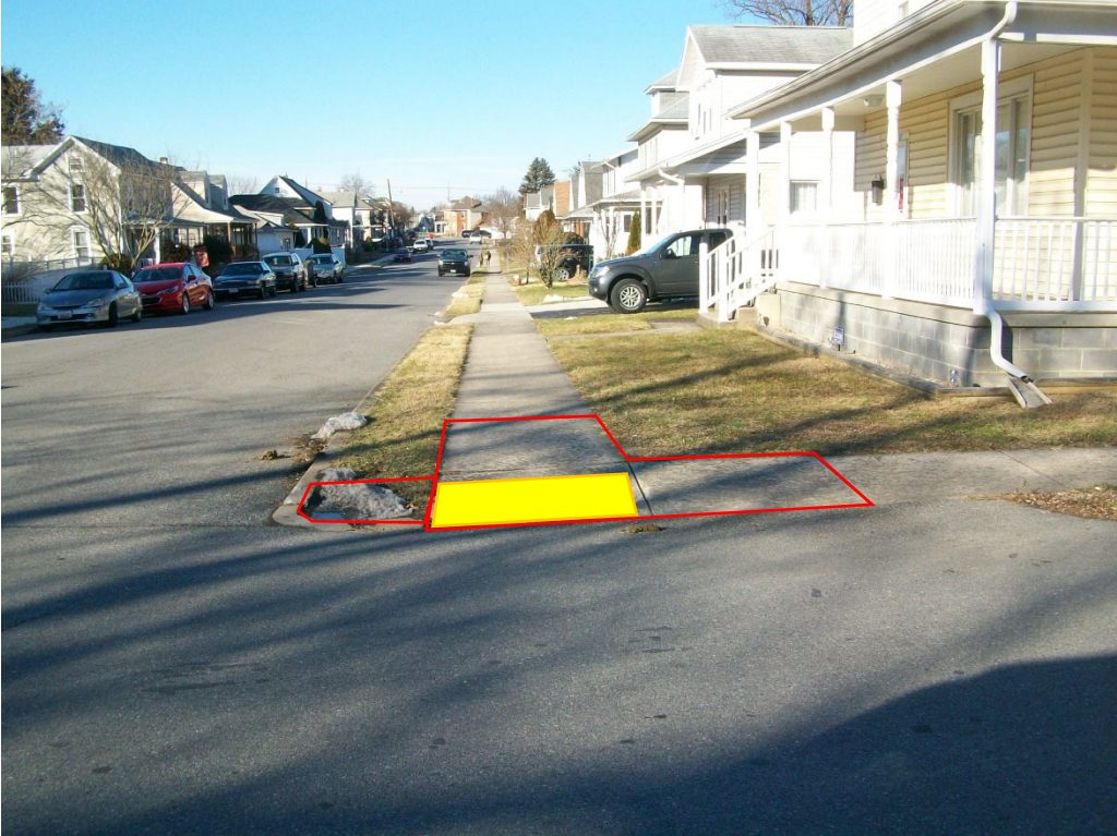
Coffman Avenue at Gay Street: Construct Parallel Ramp STD. No. MD 655.12
