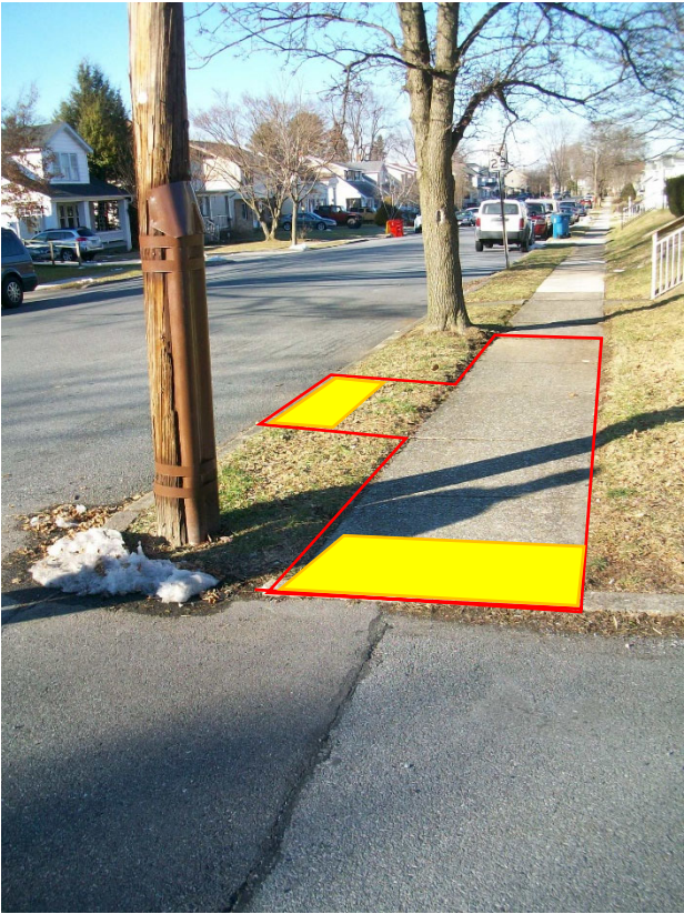
Roessner Avenue at Gay Street: Construct Parallel Ramp and Perp. Ramp
